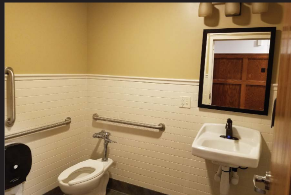
Downstairs half bathroom is ADA compliant
